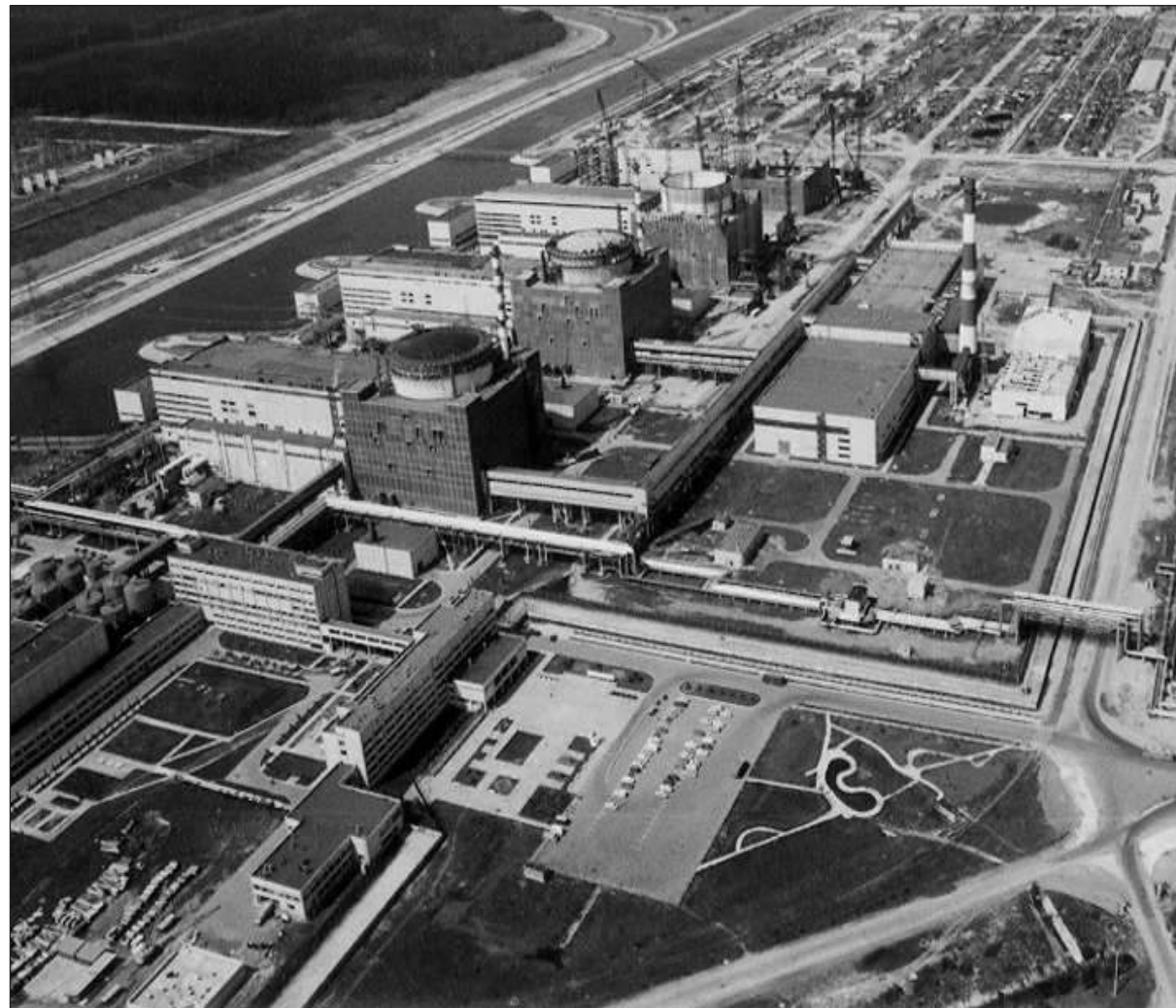
The Bushehr nuclear power facility in Iran
